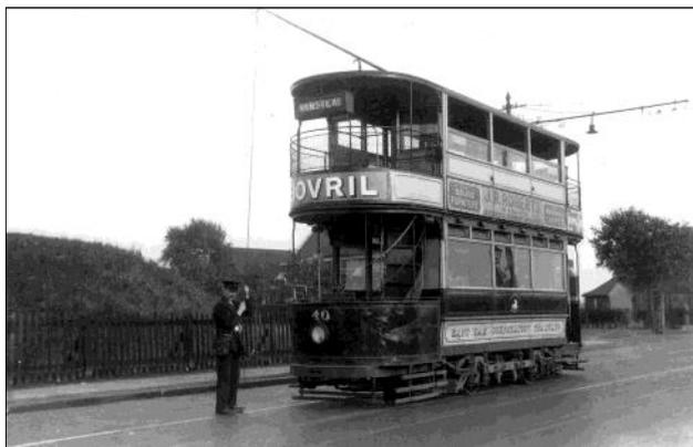
These **Ilford cars** were the last new trams to be supplied to a London system. Built by Brush in 1932 on a Peckham P22 trucks, car 37 here retained its number in LT days until sold in 1938 to Sunderland. This view is in at Chadwell Heath in 1938 and was taken by W.A.Camwell.
